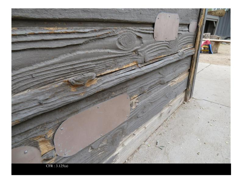
Photographer: KATIE PRICE Date and Time: 19-AUG-20 2pm Inspection No: 2016082569869258 Description: Wooden wall with protruding nail heads in goat enclosure
