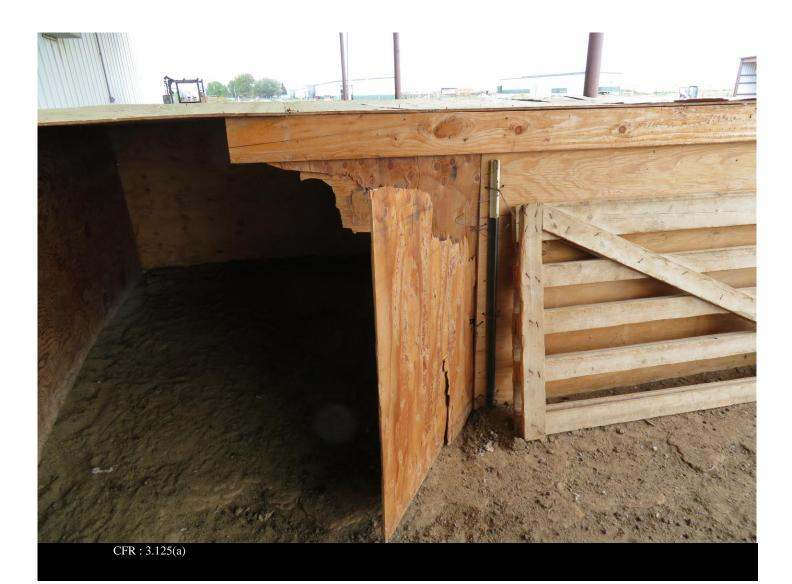
Photographer: KATIE PRICE Date and Time: 18-AUG-20 3:30pm Inspection No: 2016082569869152 Description: Broken shelter with jagged edge in sheep enclosure at Multipurpose Building
